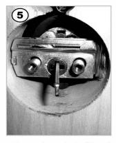
Viewed from the inside of the door the mortise cylinder is correctly located through the deadbolt as shown.
