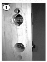
Prepare and bore the door using the template supplied and then fit the deadbolt, [top] and latch [bottom] adjusting as necessary for door handing.
