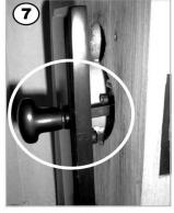
Check Deadbolt is in the un-locked position then offer up inside escutcheon locating both lever spindle and thumb piece. Thumb piece must be in the vertical position, as shown, for correct orientation of the thumb piece.
