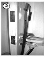
Take the exterior grip set assembly and offer up to the door ensuring that the fixing posts, the central housing and spindle are all correctly located, then push the grip set flush with the door panel.
