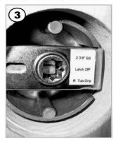
Viewed from the inside of the door the central spindle housing and the spindle are correctly located as shown.. On solid brass trim the temporary fixing of screw cover may assist in holding the grip set in position, see *figure 10*.
