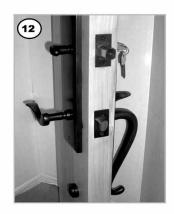
Check for alignment and operation, and tighten all fixings. On BZ trim fasten outside trim with the wood screws supplied.
