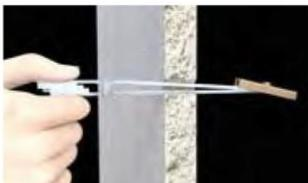
1. Slide metal channel into the pre-drilled hole
